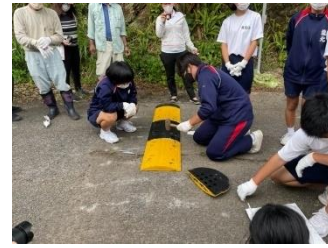
Figure 15: Installation of speed bumps by Ryukoku Junior High School in Tatsugo Town (April 2022)
