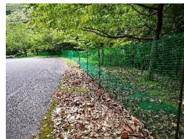
Figure 18: Animal blocking fence installed on the road in the vicinity of Mt. Yuwandake (7) on Amami-Oshima Island
