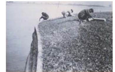
The Higashiyoka construction area at the Ariake Sea in March 1961
